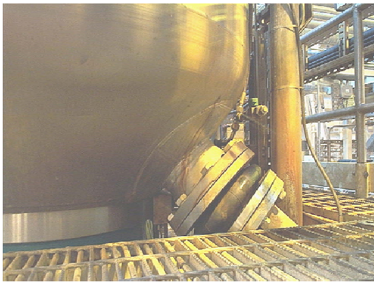
Figure 1.1 Separator OFPX717 after it has been repaired and cracked for the second time
