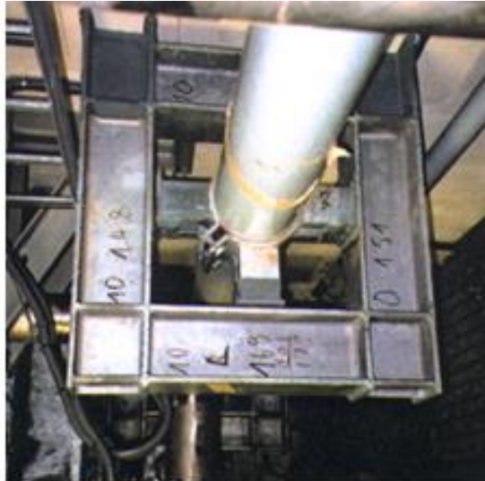
Figure 3.1: Example of a guide support in a piping system.
